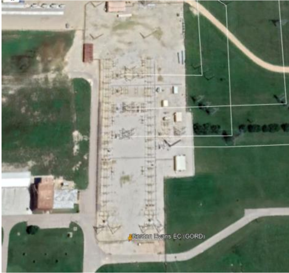
Figure 33 – Gordon Evans 138kV Substation
